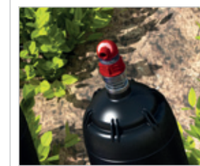
Triple effect air release valve working in air admission/expulsion also being able to eliminate the pressurized air accumulated in the pipe system.
